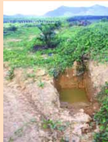
> During periods of heavy rainfall silt pits and roadside soakaways retain water and soil run-off
